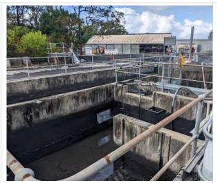
Plate 4.13 Oil water separator capturing runoff from the oil storage facilities, diesel tank storage, workshop / maintenance areas and wash bay
