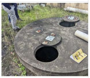
Plate 4.16 Oily water separator for compressors
