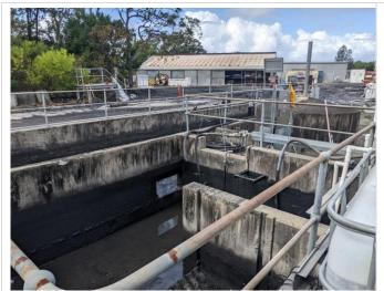
Plate 4.13 Oil water separator capturing runoff from the oil storage facilities, diesel tank storage, workshop / maintenance areas and wash bay
