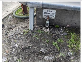
Plate 4.15 Grouted drain valve, removing ability to drain diesel storage bund, in accordance with the EPL
