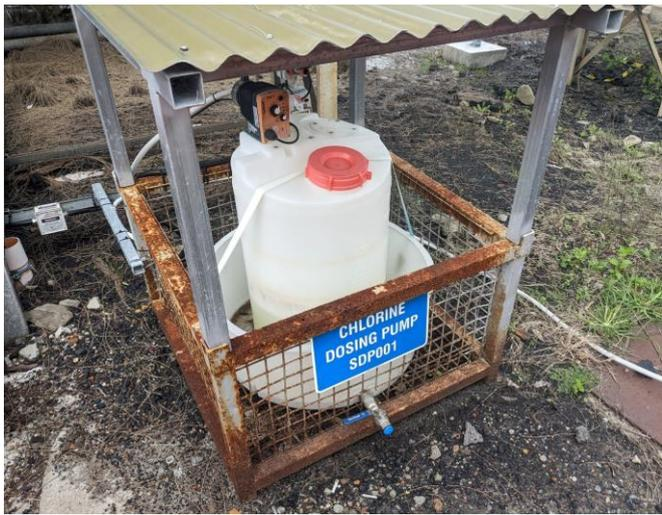
**Plate 4.7** Chlorine dosing pump
