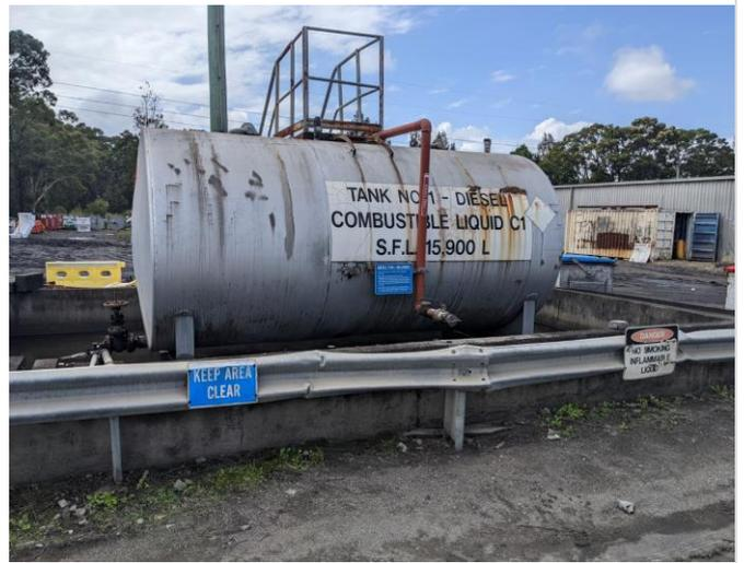
**Plate 4.8** Above ground, bunded diesel storage tank
