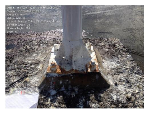
Photo 3. Current condition of the marker fixing to the concrete block
